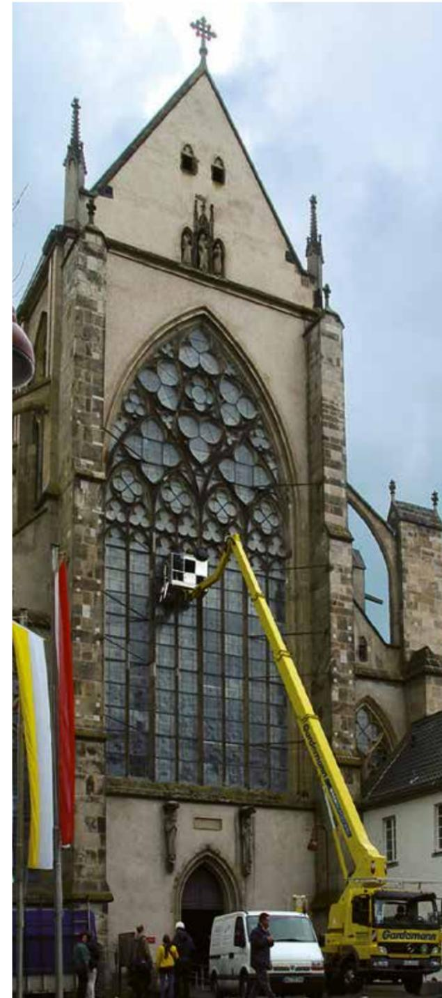
Attaching the glass sensors to the outside of the protective glazing
