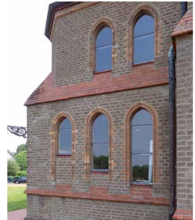
Closure of the building envelope by the protective glazing - the art glazing is simply placed in front from the inside after restoration.
