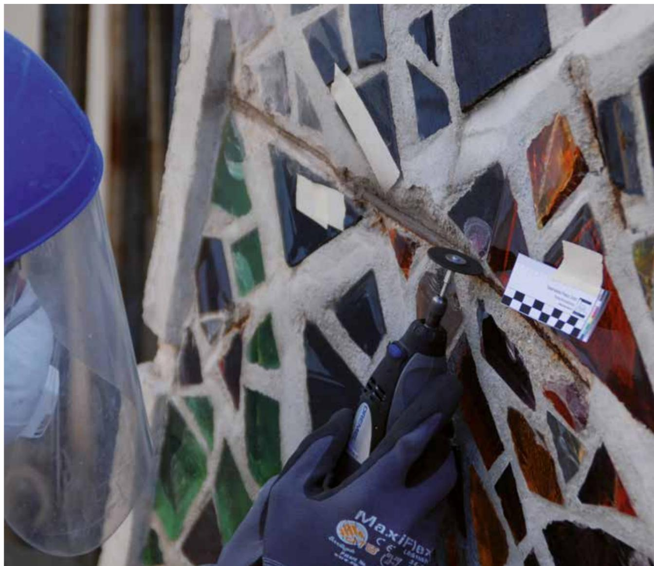
38 Exposure of the corroded reinforcement bars - Neustadt am Rennsteig
